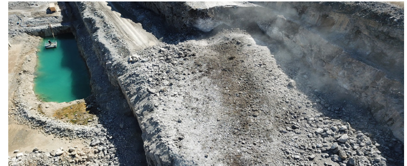
Post Blast photo of the first shot
