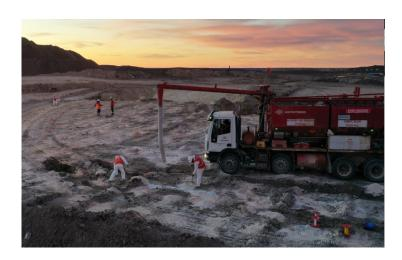
Hydromite 100 is a booster sensitive emulsion explosive which is produced on site by sensitizing an emulsion matrix by chemical gassing. Hydromite 100 is pumped directly into the borehole by an approved pump truck or pump unit.
