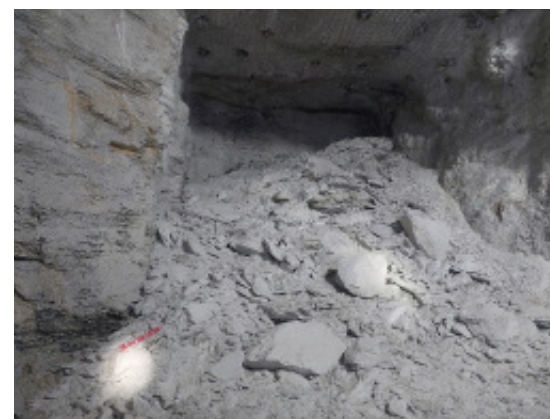
Fig. 5: Pattern underground: drilled face as basis for IMAGE TRACER and AUTOCAD
